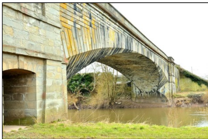
Over Bridge from Alney Island, linking Cheltenham Road and Highnam
